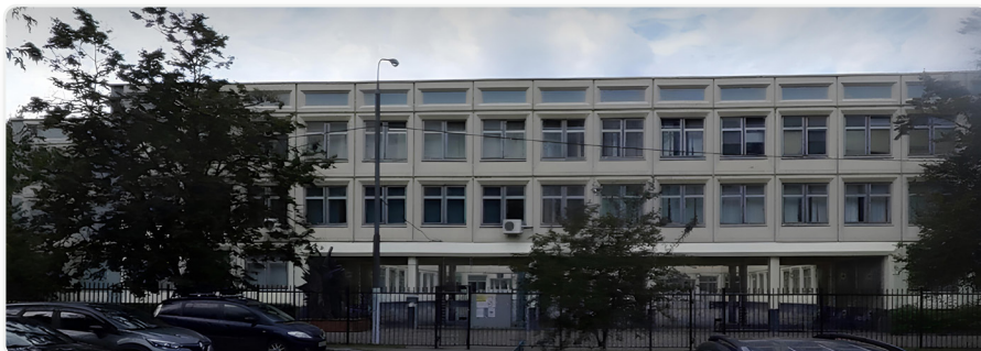
Fig. 1 Three-storey school in Ivanovskoye District, Moscow
