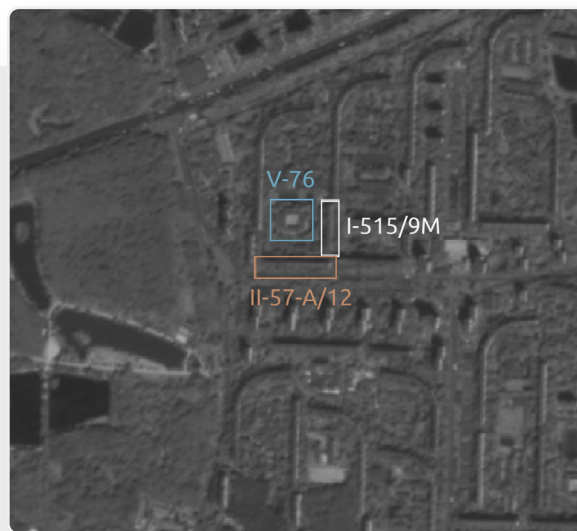
Fig. 5 Buildings in a space image
