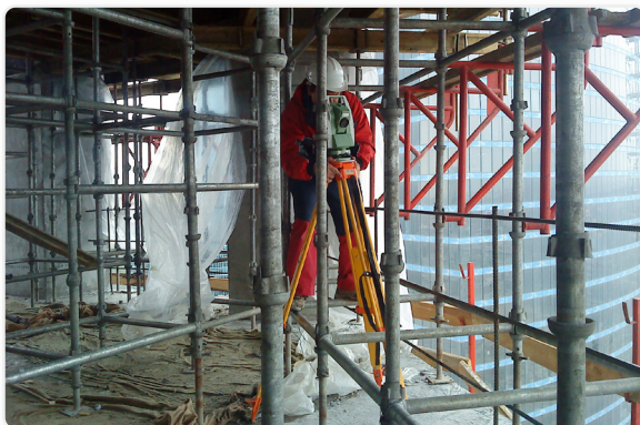
Fig. 6 Working area of monitoring on the mounting horizon: real-world examples (Vladimir A. Zubarev's personal photos)
